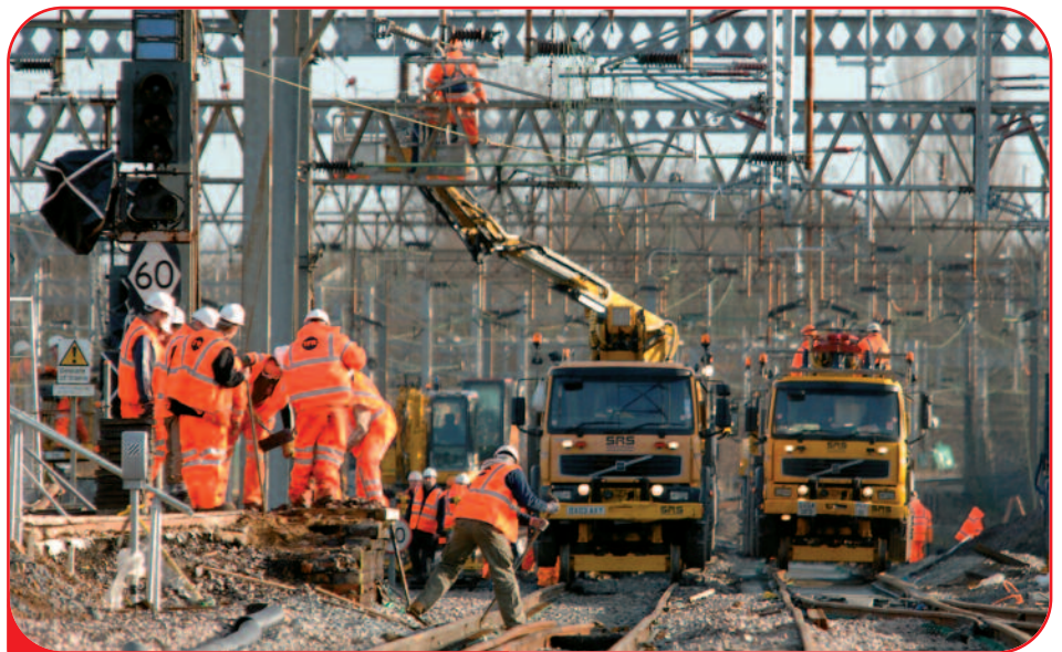
Engineers work to upgrade the line
